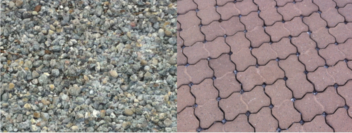
Figure 3 – Porous Concrete (at left), Paver Stones with Gravel Infill (at right) (Photo by S. Trinkaus of Cincinnati, Ohio LID Demonstration Project)
