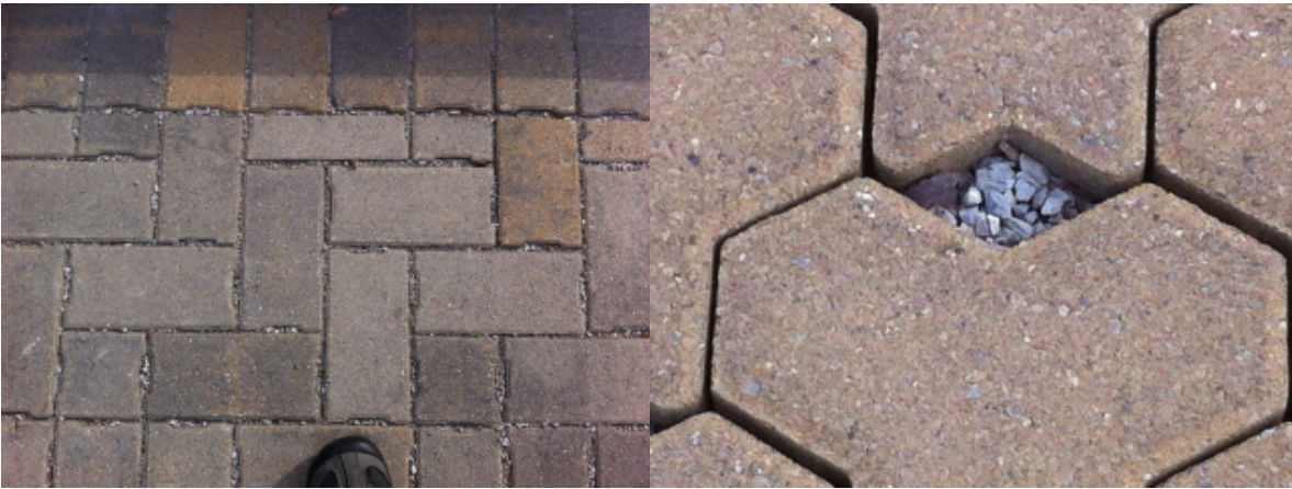
Figure 4 – Paver Bricks with Coarse Sand Infill (at left) and Ornamental Pavers with Stone Infill (at right) (Photo by S. Trinkaus of Cincinnati, Ohio LID Demonstration Project)
