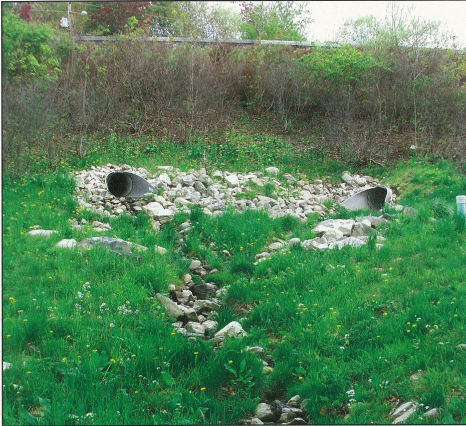
Outlet pipes from existing state and municipal drainage system discharges at the southern end of the City Meadow.
