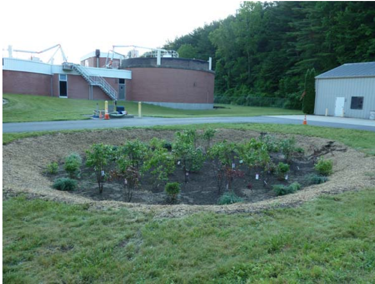
Figure 4 - Bioretention System (Trinkaus Engineering, LLC)
