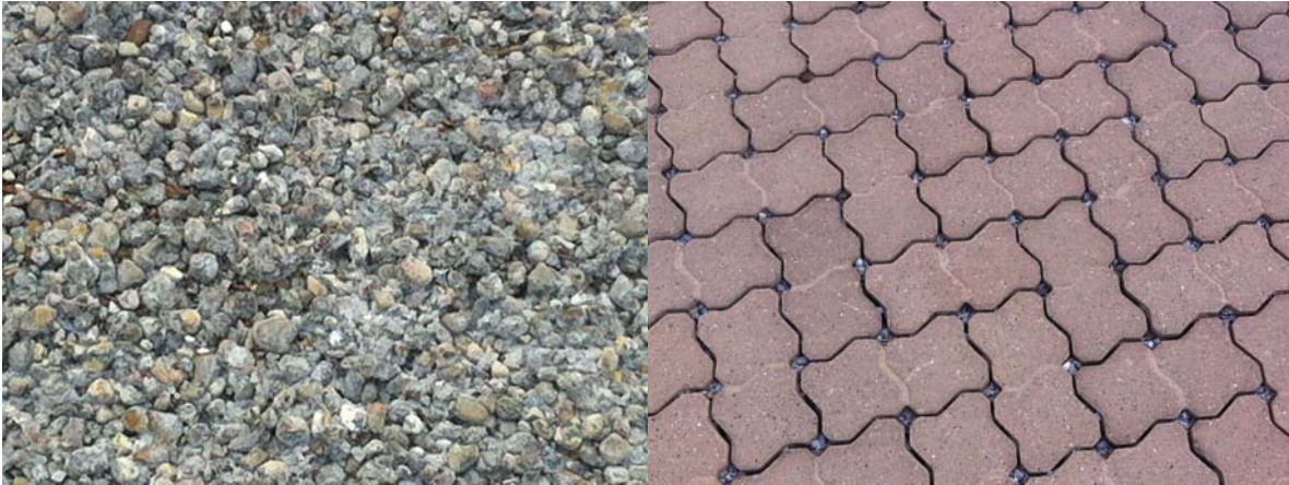
Figure 6 – Porous Concrete (at left), Paver Stones with Gravel Infill (at right) (Photo by S. Trinkaus of Cincinnati, Ohio LID Demonstration Project)
