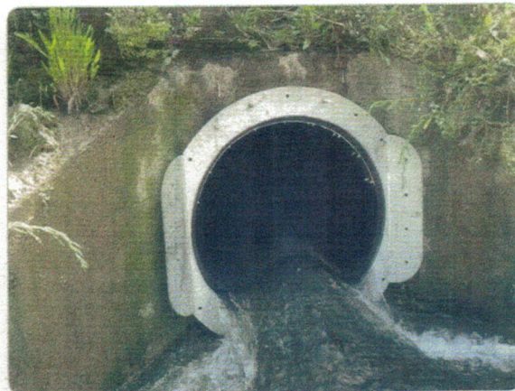
WASTOP® - 100% backflow prevention with low headloss. Giving you peace of mind.
