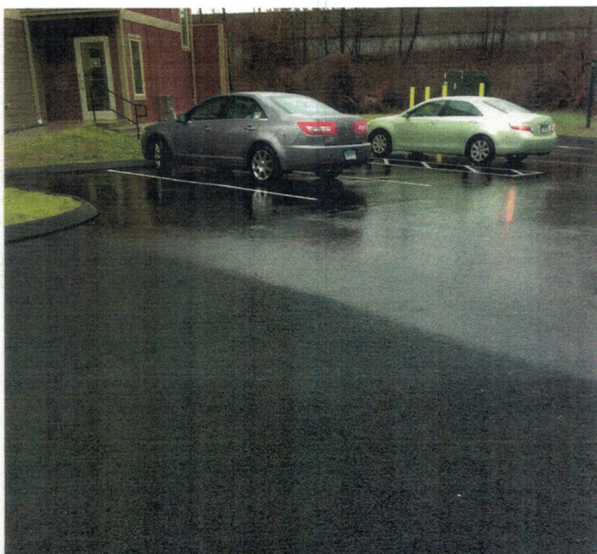
Figure 8. During a rainfall event, permeable pavement (foreground) and standard pavement (further back) show very different levels of drainage.
