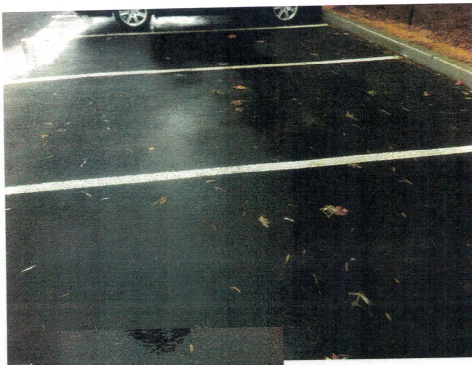
Figure 5. A partially failed permeable-pavement system became clogged and simply discharged water at the bottom.
