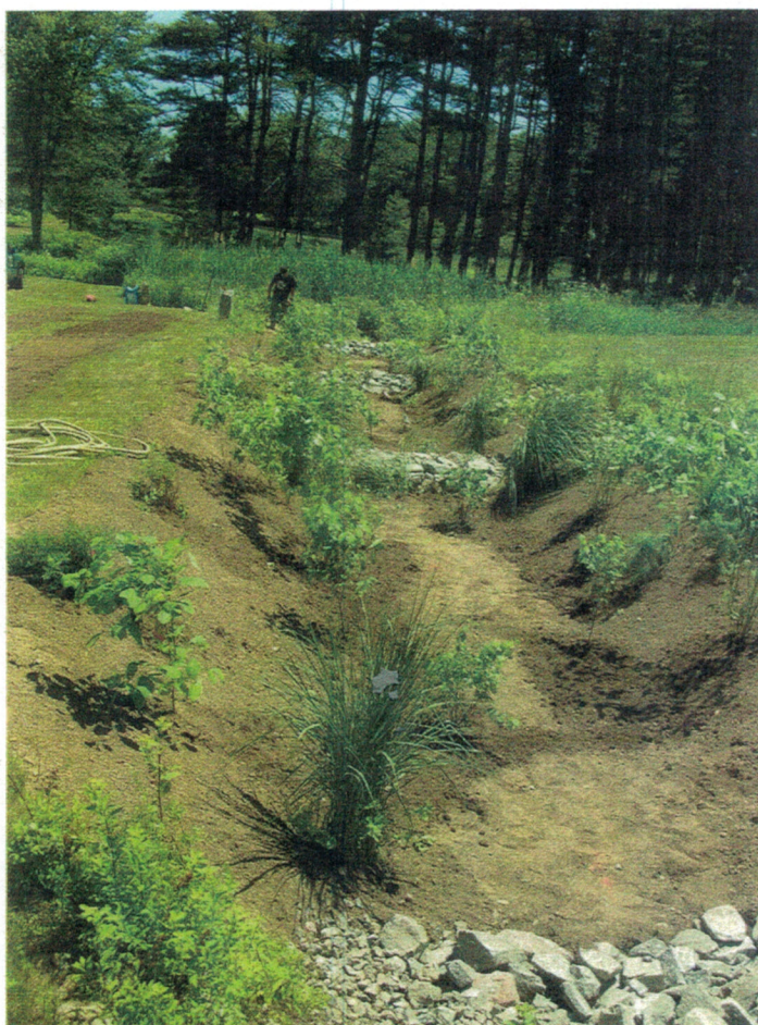
Figure 7. A bioswale demonstration project replaced riprap swale at the outlet of a drainage pipe.
