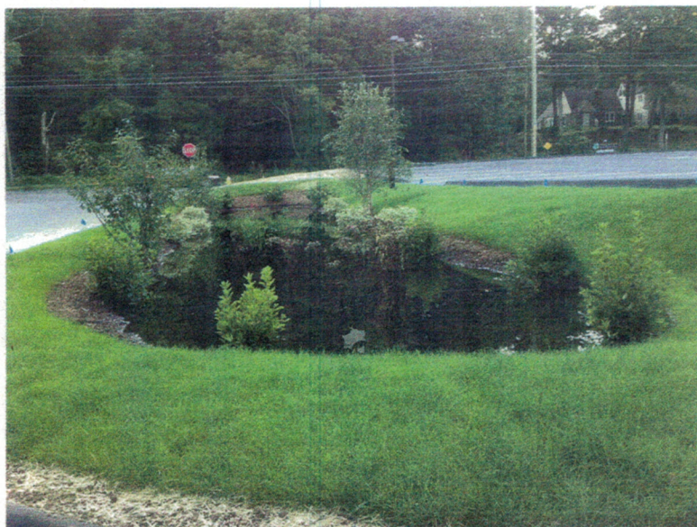
Figure 3. Another ineffective rain garden was installed above previously filled wetland soils.
