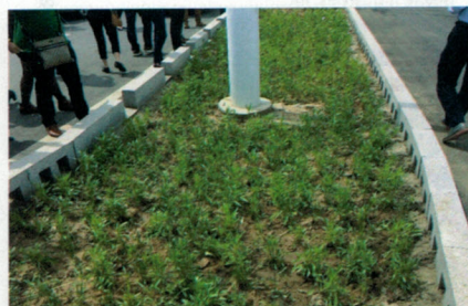
Figure Three - Bioswale along new roadway
