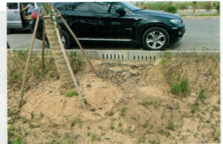
Figure Four - Bioswale with erosion at the inlet, resulting in sedimentation at the bottom.
